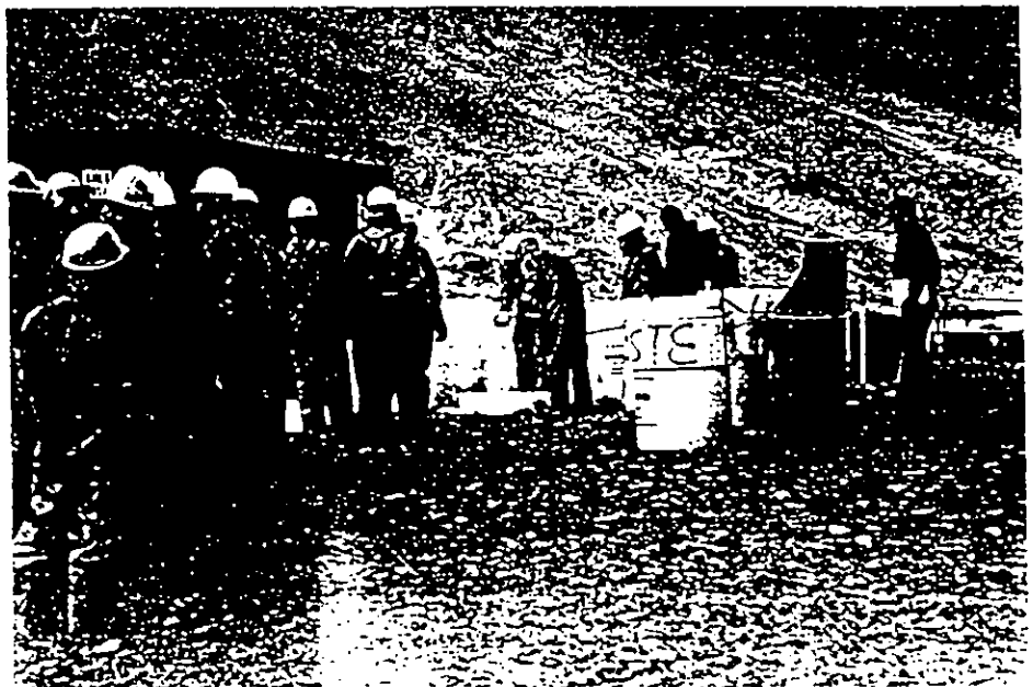
Workers in protective gear stand in a line on a construction site, likely related to the hazardous waste cleanup at Saint Lawrence Island, Alaska.
